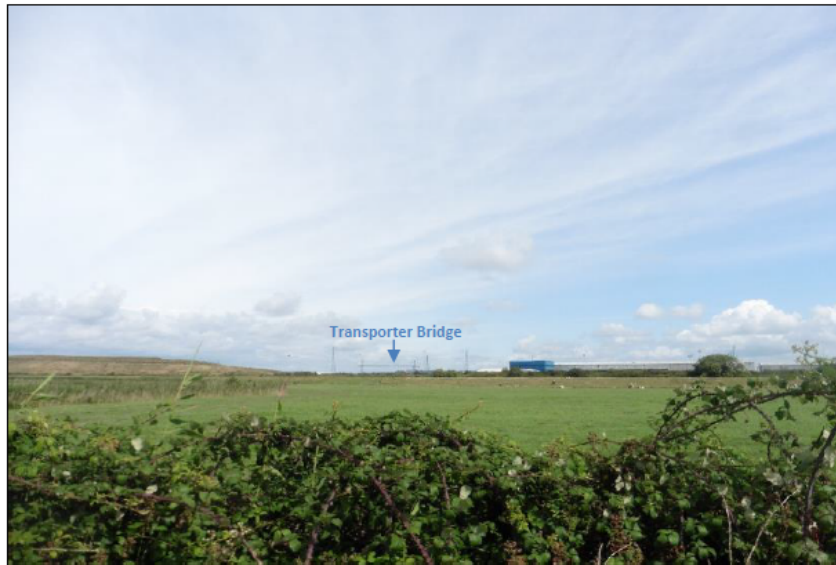
Plate 6: View north-east towards the Transporter Bridge from the WCP further north than plate 5. Site to right of photo.
